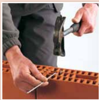
Install wall ties
