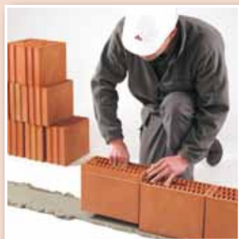
First course bedded in normal mortar
