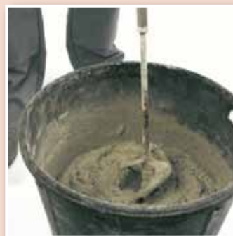
Mix only enough Porotherm bed joint mix
